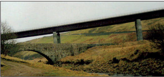
Road bridges old and new at Dunbeath.
