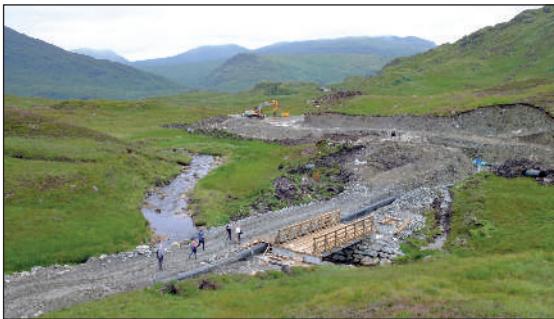
One of the new run-of-river hydro schemes in Glen Falloch under construction, within the Loch Lomond and The Trossachs National Park.
