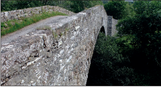
The Wade bridge at Daviot.
