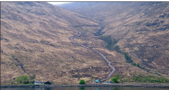
A new run-of-river hydro scheme being built at Kingairloch.
