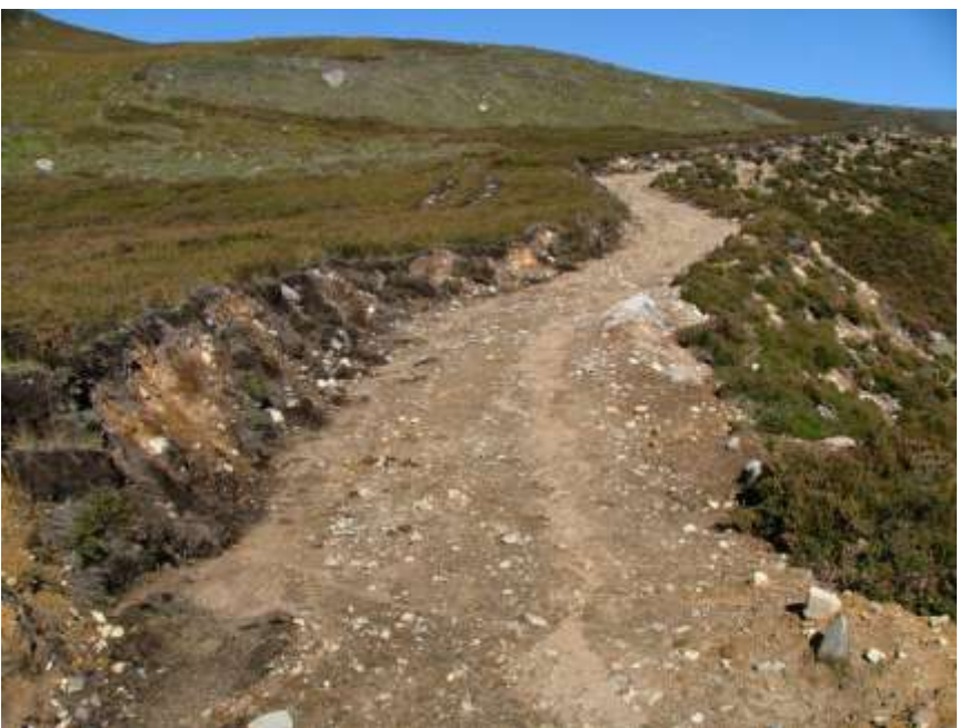
Above: Bulldozed track without drainage, Invercauld Estate
