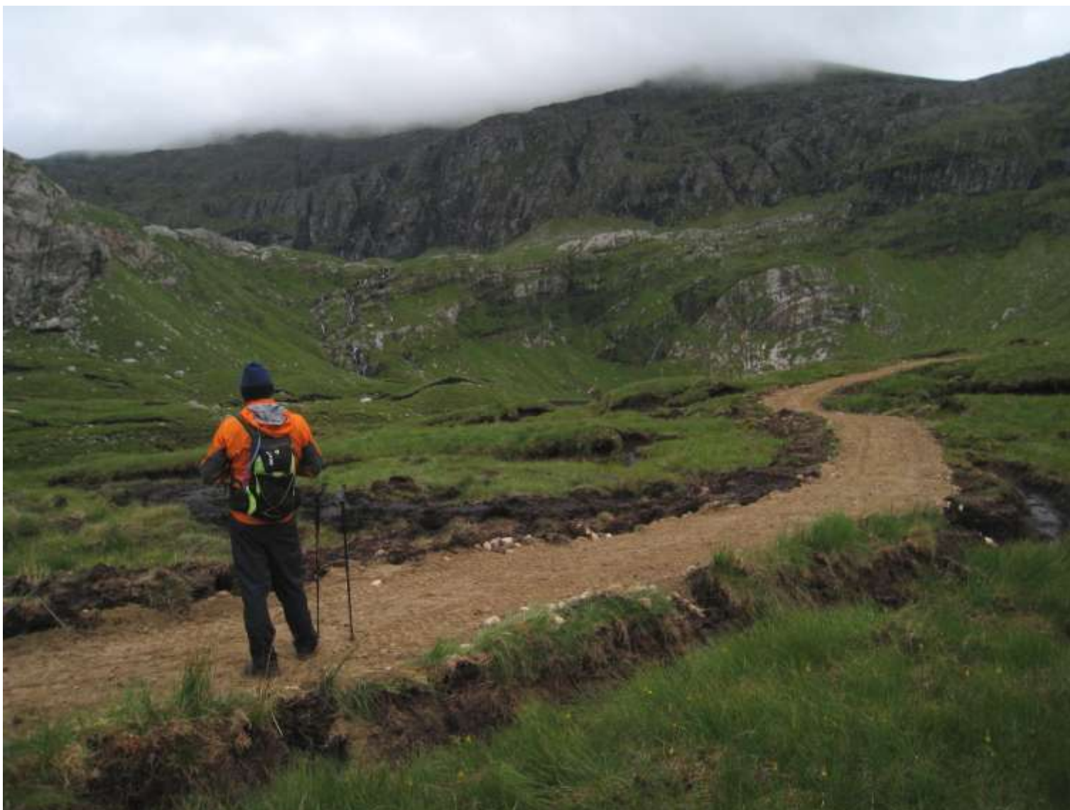
Photographs: Top: A section of track crudely excavated out of peat and already eroding. Bottom: Track running through peat bog.
