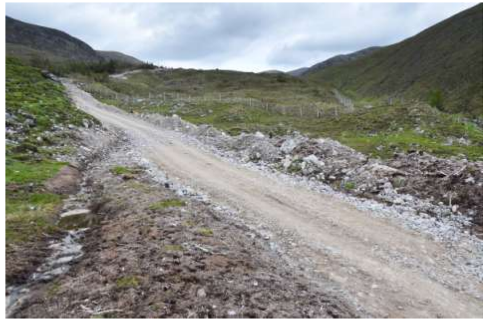
Above: Poorly constructed track by Loch Monar
