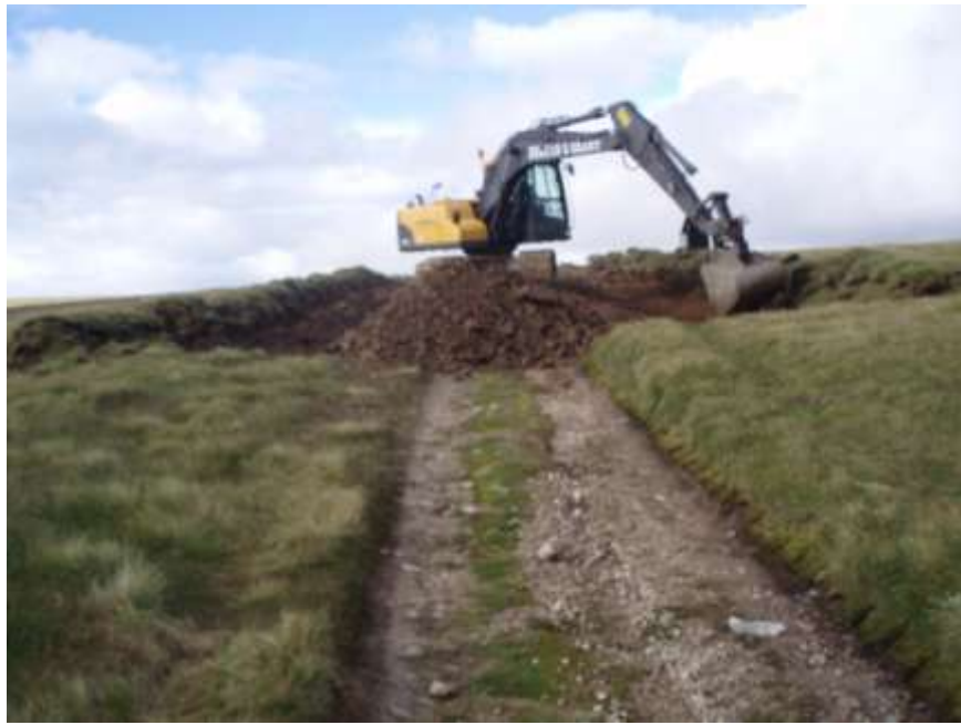
Below:, left and right: track upgrading at Glen Feshie
