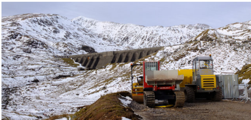
Development in the high mountains, here the dam for the pumped storage scheme below Ben Cruachan. Renewable energy schemes, however well-intentioned, have a major impact on wild land whether or not formally designated as a Wild Land Area
