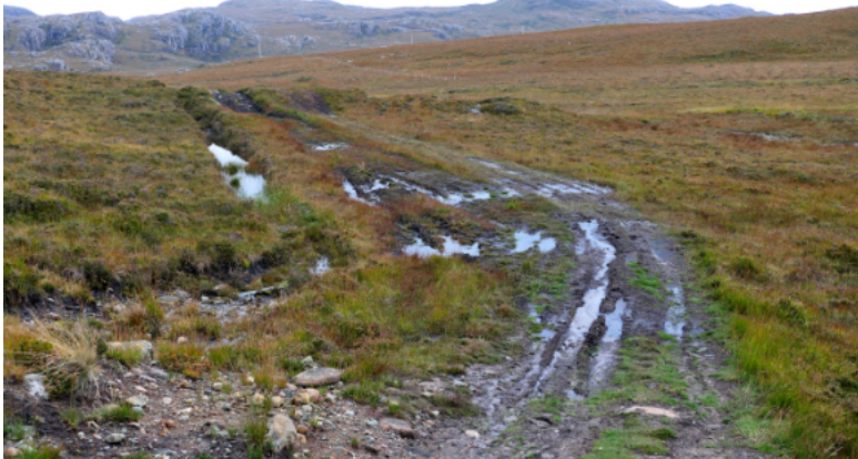
Below: The access to the mast on Cliff Hill, Poolewe, Wester Ross. Photo. James Fenton
