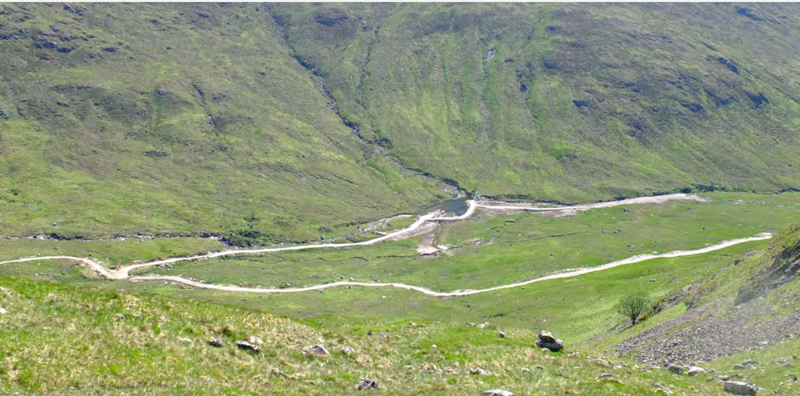
Bottom left: A new dam on a previously wild loch within the Wester Ross National Scenic Area.
