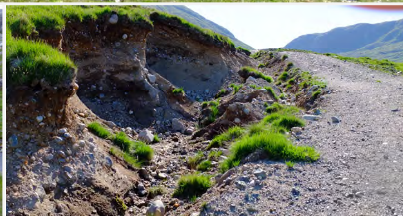
Bottom right: A new track already showing significant erosion. The construction style of this track can only be described as 'shoddy'. All hydro schemes necessitate access tracks. In Scotland's wet climate, these are likely to erode unless extremely well built, with continual clearance of cross-drains and pipes (something that rarely happens in my experience).
