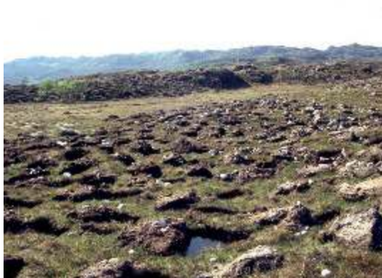
Close-up of mounding for tree planting at Inveralligin. Such mounding allows trees to be established in places they might otherwise be unwilling to grow. Such planting schemes also involve the construction of deer fences.
