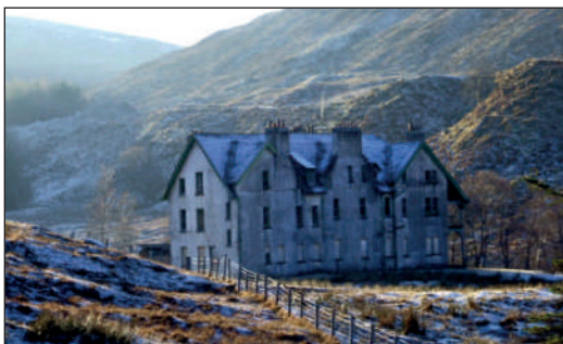
Sron na Larig Lodge shooting Lodge in the Monadhliath (recently demolished).
