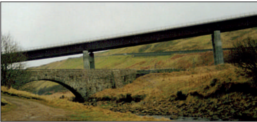
Road bridges old and new at Dunbeath.
