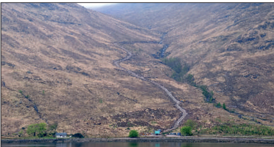
A new run-of-river hydro scheme being built at Kingairloch.
