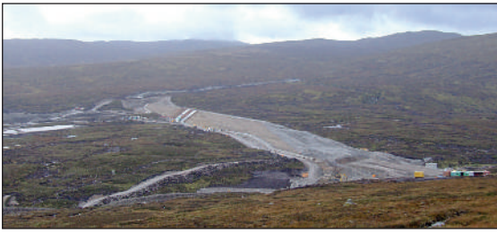
The new Glendoe pumped storage scheme. This shows the dam under construction to create a high altitude reservoir (over blanket peat).
