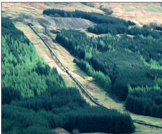
A modern Highland landscape north of Loch Tay showing a hydro pipe, tailings from a hydro tunnel and commercial forestry plantations.
