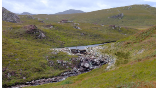
The Boor Burn in Wester Ross where you could enjoy a wild walk up to the moorland above (left). Now you encounter a new path and a concrete dam.
