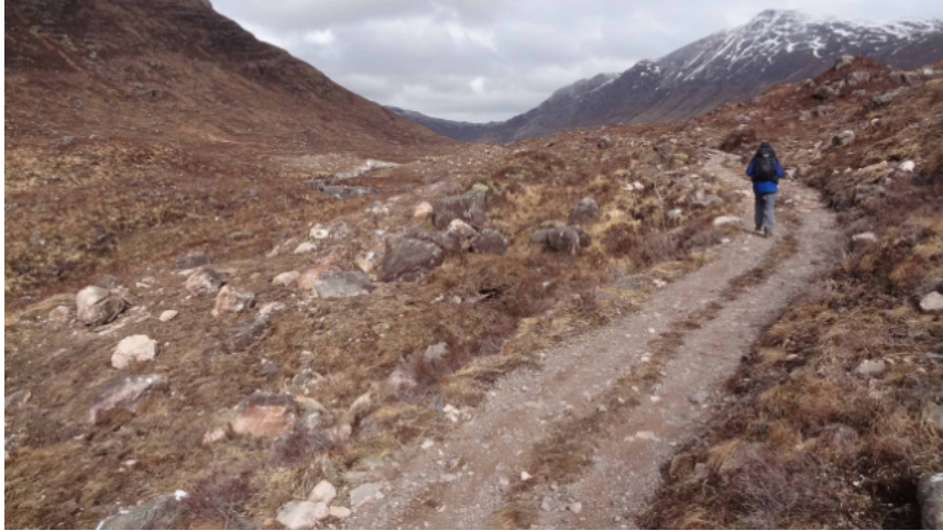
The Coulags scheme, Glen Carron. Top marks here! The intake weir is well sited outwith the glen proper (they could have been greedy and gone further in for a bit more 'fall'); the access track to it is beautifully restored, and looks like the old stalker's path has just been widened a bit for quad vehicles. Photo. David Jarman
