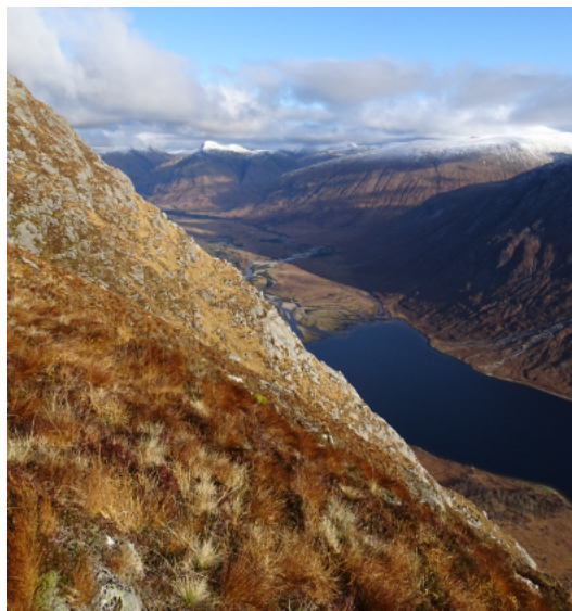
The head of Glen Etive from Beinn Trilleachan. The hydro-schemes are on the side glens to the right.
