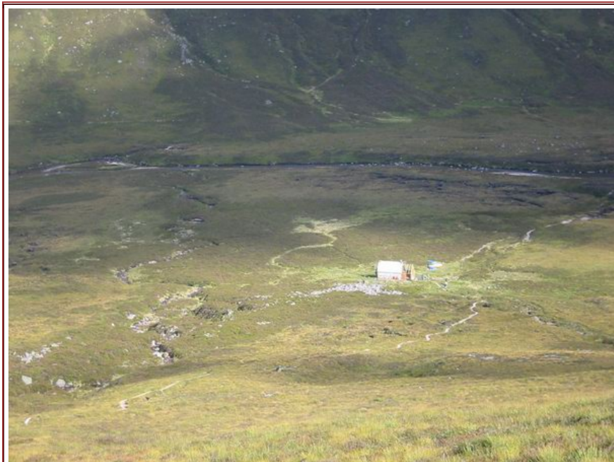
Corroul Hut, Lairig Ghru with the toilet in construction.
