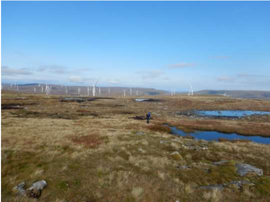
Figure 3.15 Stronelairg wind farm looking north from Creag an Dearg Lochain (813m)
